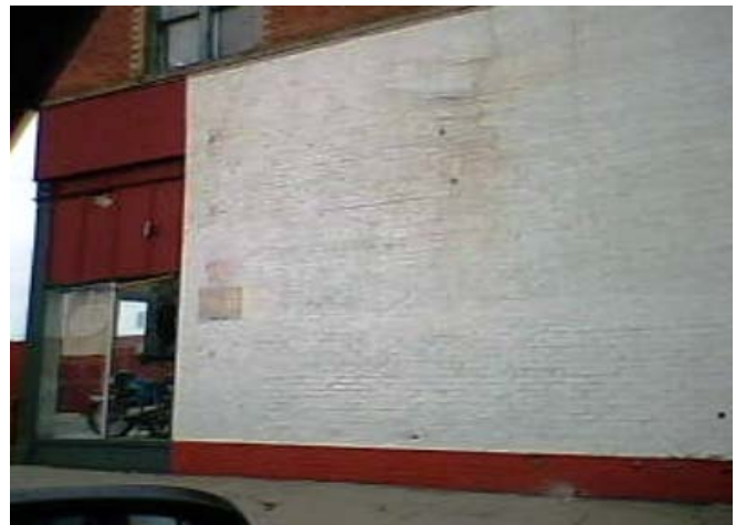
Project wall before
